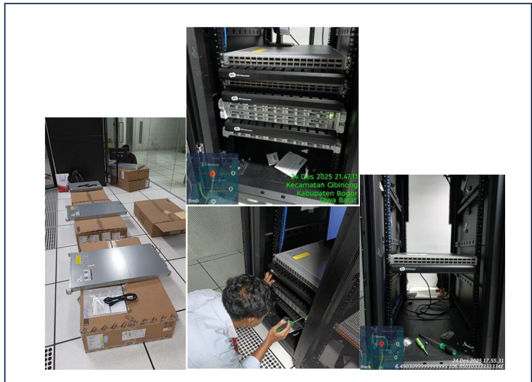
Gambar 5 Empat unit Cisco (APIC, Spine and Leaf) - 23 Desember 2025
